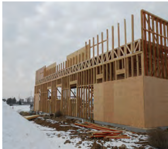
Figure 43—Wall bracing
