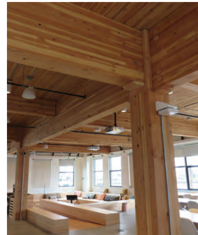
Figure 38—Beam column connection
